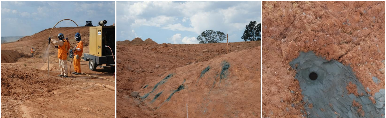
Figure 2. Treatments carried out in excavations with canaliculi
